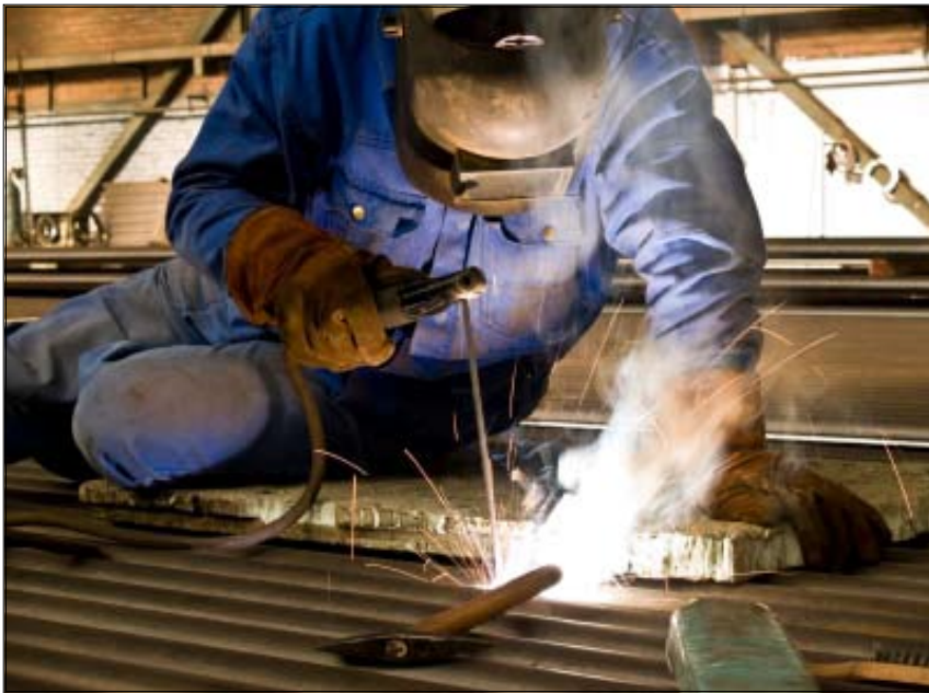
Shielded Metal Arc Welding (SMAW)
